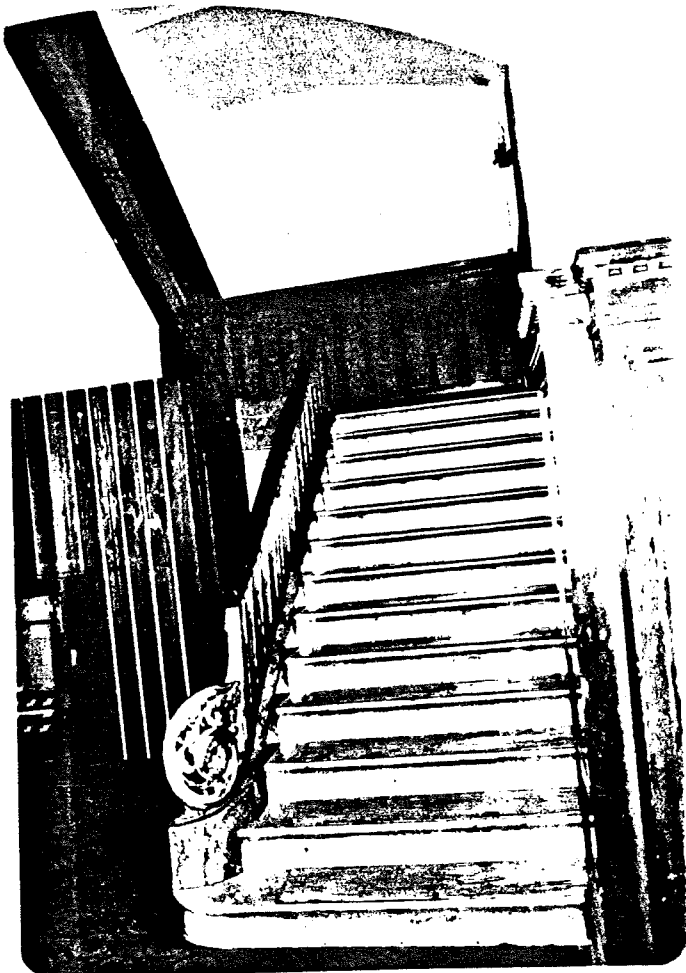
II.1.4.(a) ORIGINAL MAIN STAIRCASE
