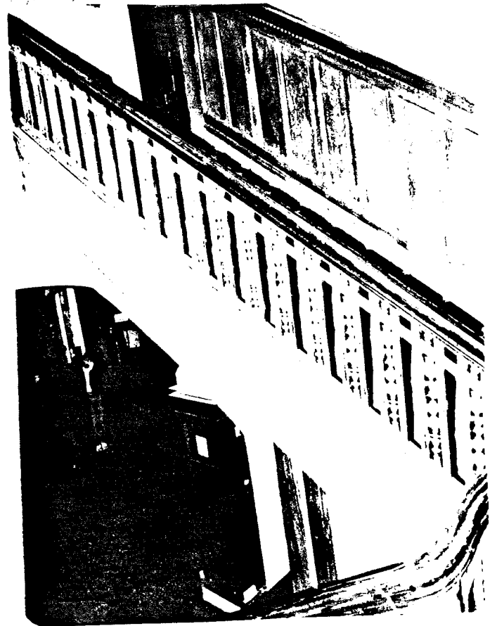
II.1.4.(b) ORIGINAL MAIN STAIRCASE WITH IRON BALUSTERS
